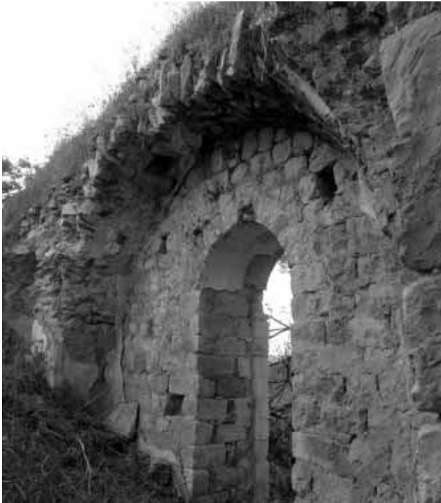
The remains of a village house partially demolished.
