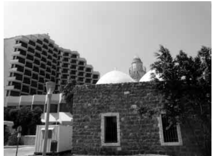
A village mosque with the Sheraton hotel in the background
