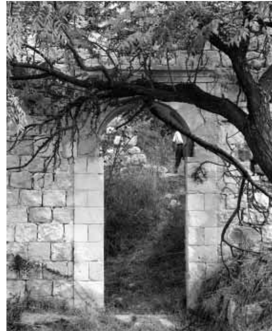
The remains of a village house partially demolished.
